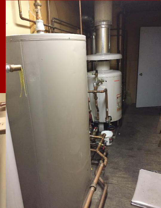
Old Hot Water Tank and Boiler
