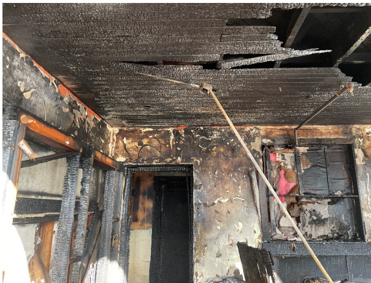
Photograph 11: 3 rd Floor Framing Damage
