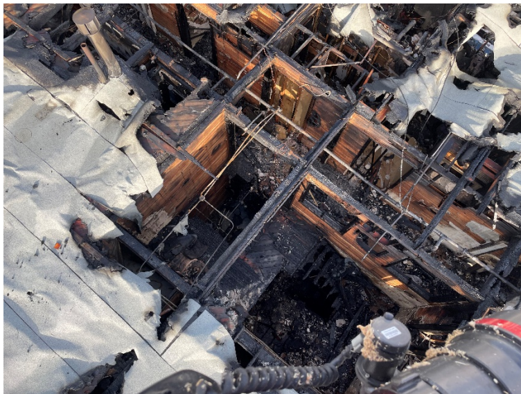
Photograph 9: Roof and 3 rd Floor Damage at Stairwell
