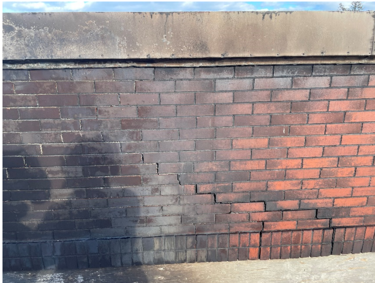
Photograph 7: Wall Facade Step Cracking
