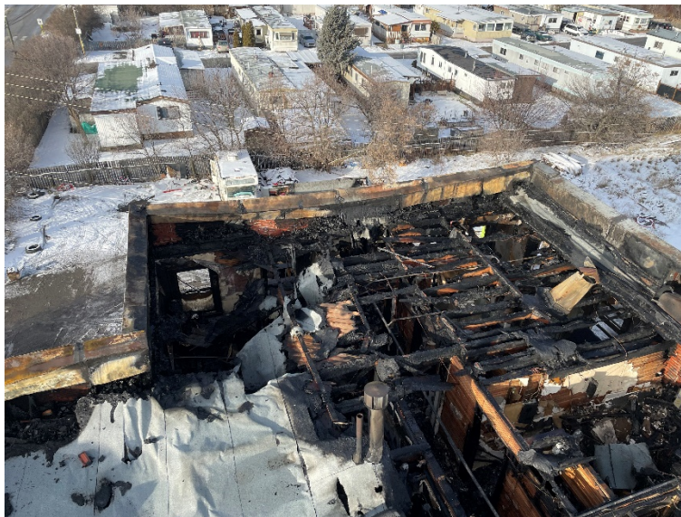
Photograph 5: Damaged and Collapsed Roof Components
