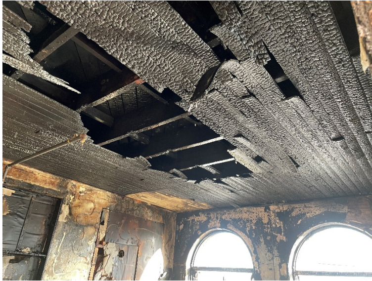
Photograph 10: 3 rd Floor System Damage
