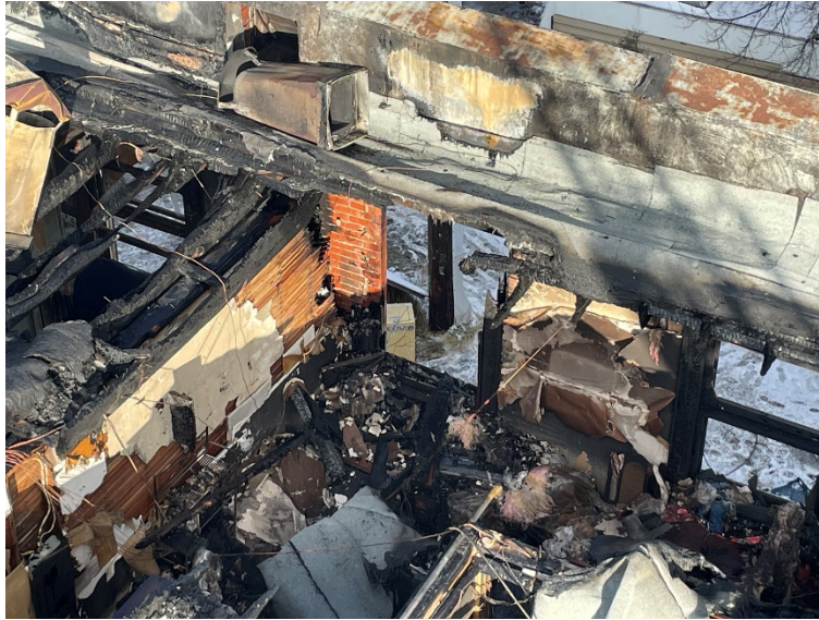
Photograph 8: Exterior Wall Damage
