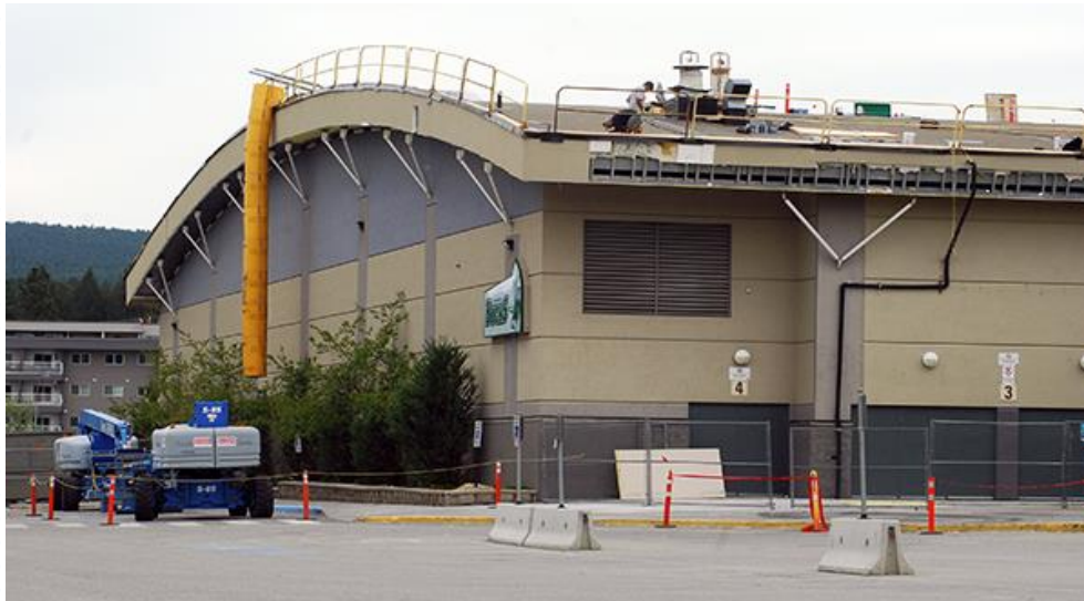
Western Financial Place Roof Replacement
