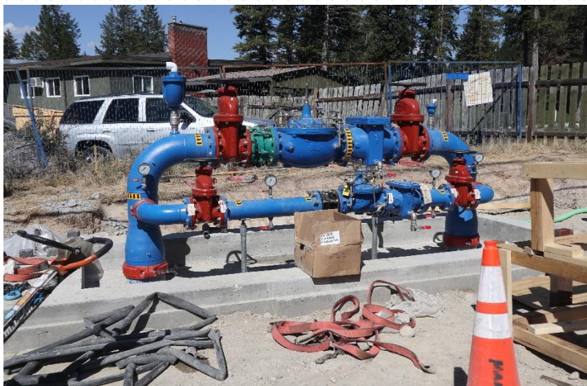
PR Station #5 Replacement
