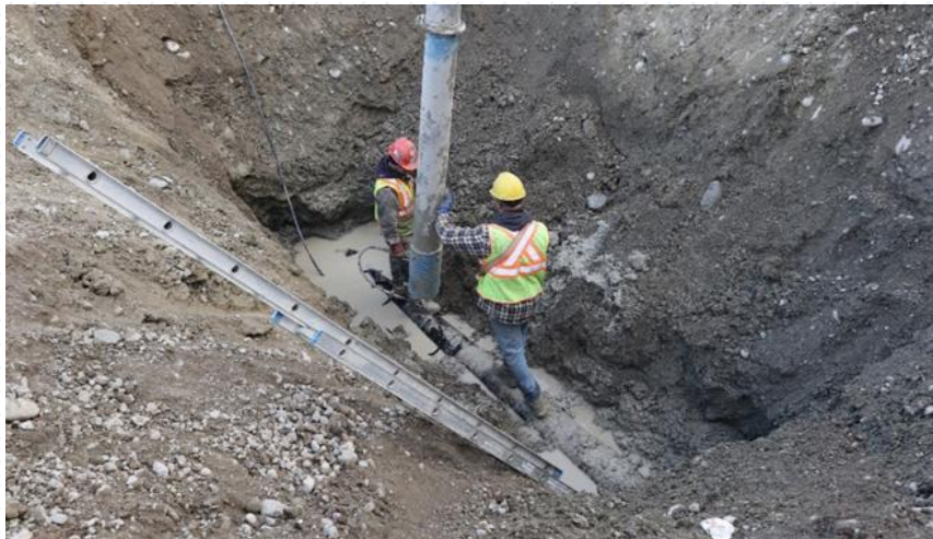
Water Main Repair Wildstone Drive
