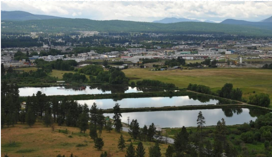
Wastewater Lagoons – North end of Cranbrook
